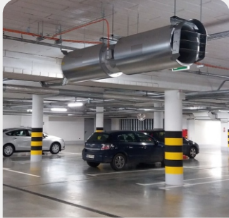
BASEMENT CAR PARKING
